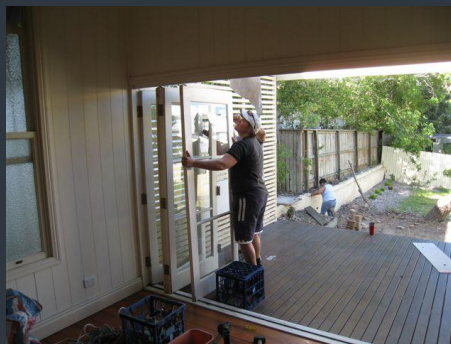
Removing Bifold Doors
