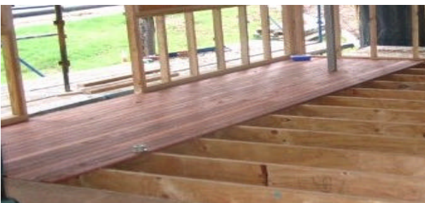
Recycled timber decking at Sustainable Home Brisbane
